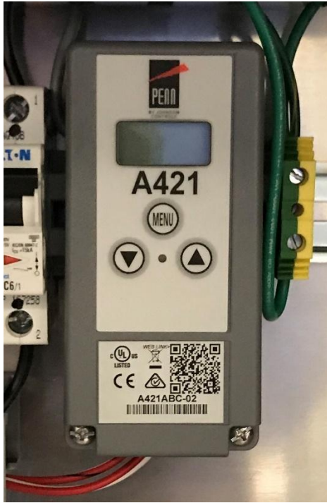
Fig. 39 Temperature Sensor Control Panel
