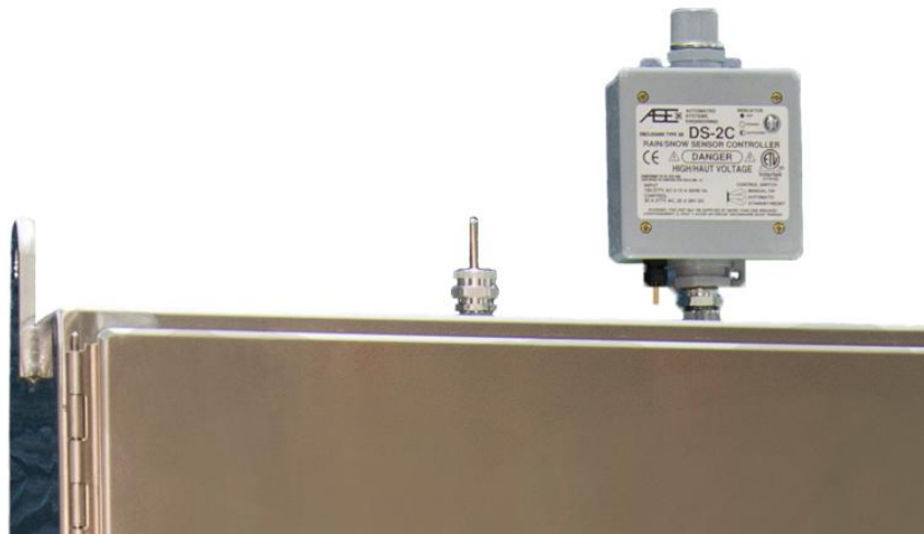
Fig. 3 Top of Control Cabinet, with Johnson Controls Temperature Sensor (left) and Snow Sensor (right)
