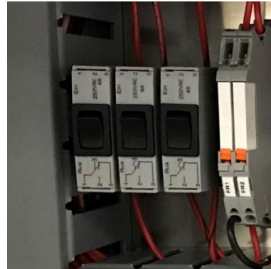
Fig. 21 Ground Fault Reset (left) and Ground Fault By-Pass Switches (right) for each of two circuits
