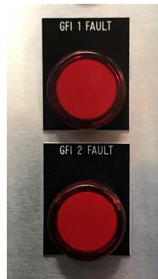
Fig. 12 GFI Fault Lights
