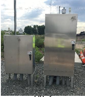
Fig. 2 1 – 6 Circuit (left) and 7 – 12 Circuit (right) Cabinet Models
