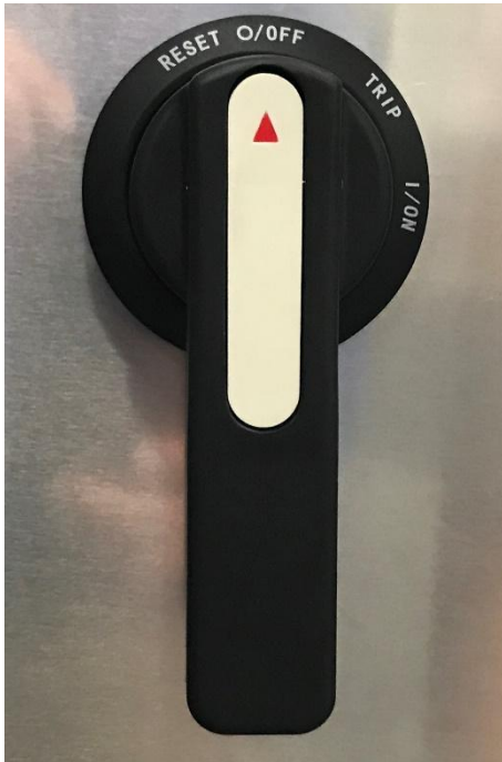
Fig. 9 Main Breaker Switch
