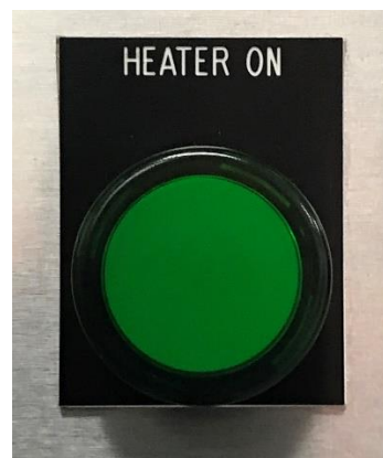
Fig. 11 Heater On Indicator
