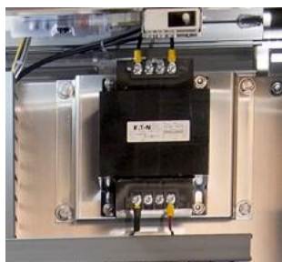
Fig. 22 Control Power Transformer
