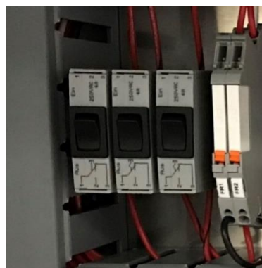
Fig. 41 Ground Fault Reset (left) and Ground Fault By-Pass Switches (right) for each of two circuits
