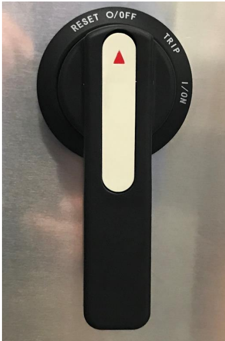
Fig. 9 Main Breaker Switch
