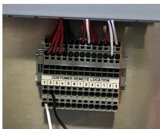
Fig. 23 Customer Connection Terminal Block
