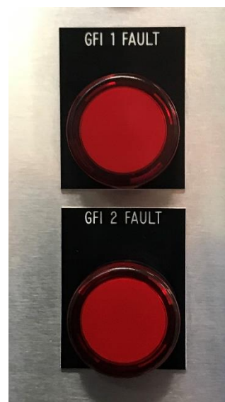
Fig. 12 GFI Fault Lights
