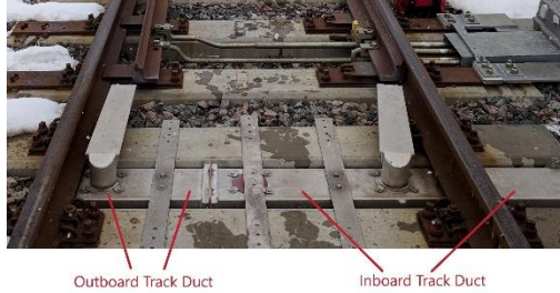
Fig. 303 Track Duct Assembled at Switch Point
