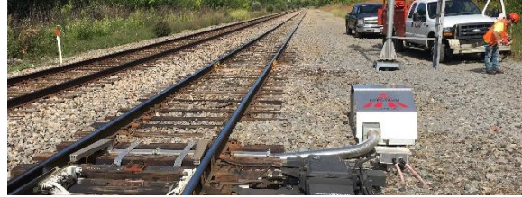
Fig. 1 RRSHA Hot Air Blower Installed at Track Site
