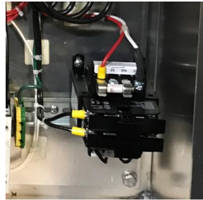
Fig. 10 Control Power Transformer
