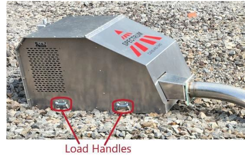
Fig. 268 Main Housing Unit Installed on Ballast Surface
