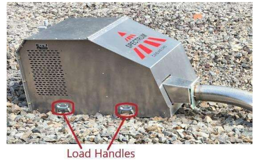
Fig. 268 Main Housing Unit Installed on Ballast Surface
