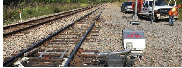
Fig. 1 RRSB Hot Air Blower Installed at Track Site
